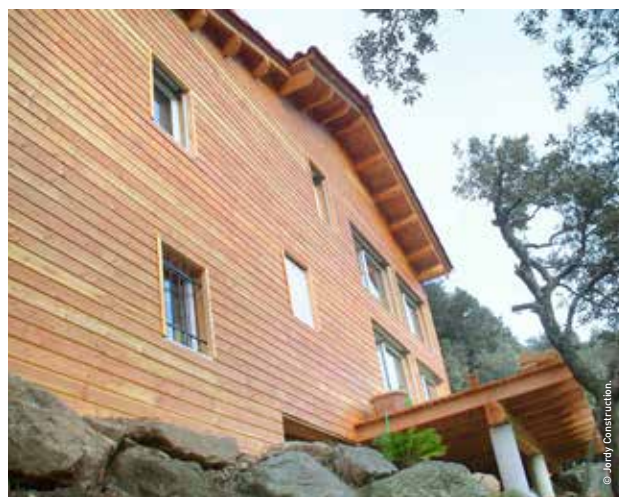
Douglas fir cladding without finish after construction.
