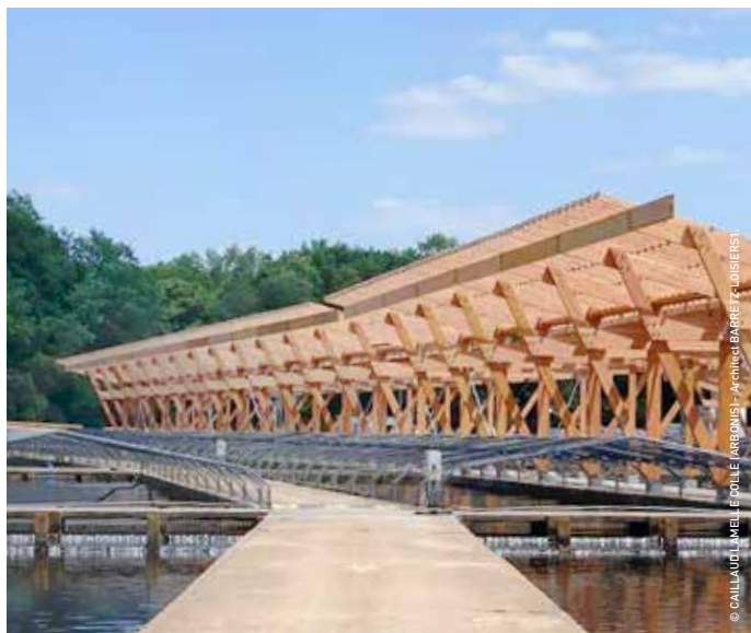
The Mézos fish farm in Landes showcases the potential uses of Douglas fir in exterior structures.
