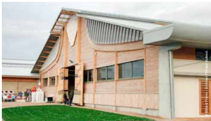
The Pôle international du Cheval (horse riding venue) in Deauville is one example of the possible uses of Douglas fir for exterior cladding.
