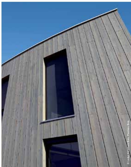
Cladding with finish (semi-transparent glaze).
